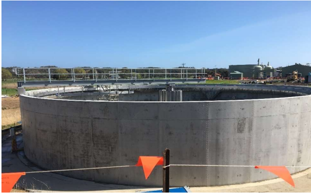
Clarifier 1D – Concrete works completed.
