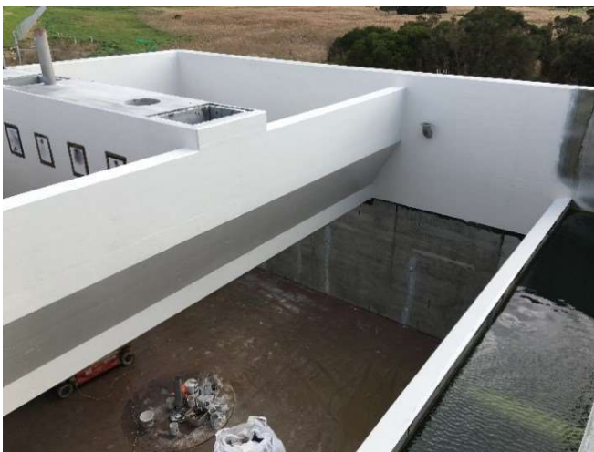
Epoxy Coating the Primary Settlement Tanks
