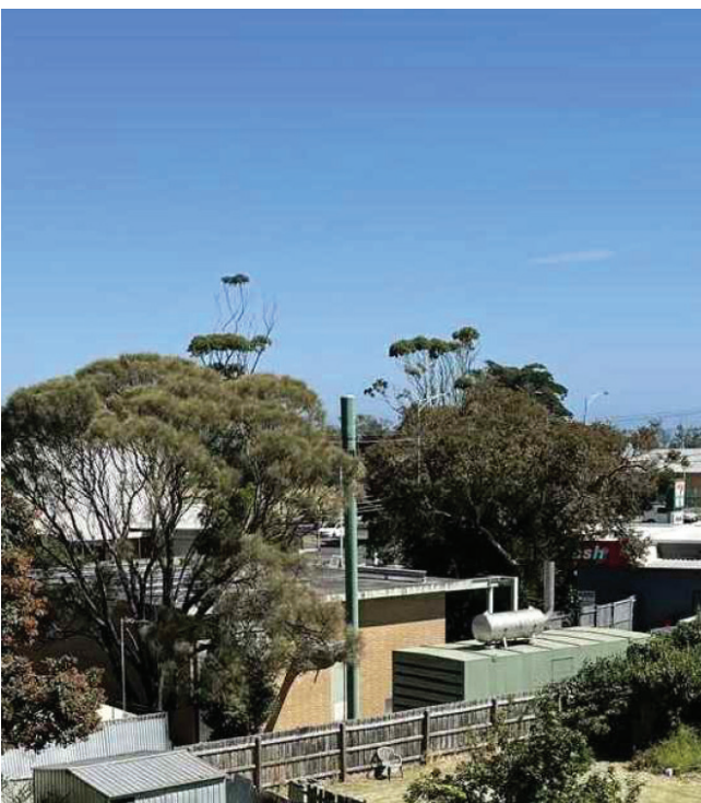
Existing stack viewed from south-east of the pump station.
