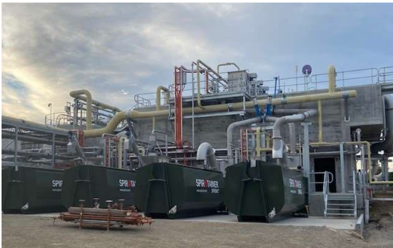
Above: Completed inlet structure.
