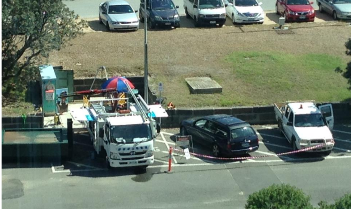
Figure 5: Facility set out during pump removal works
