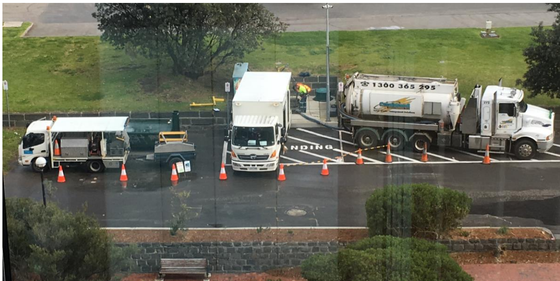
Figure 7: Facility set out during wet well cleaning
