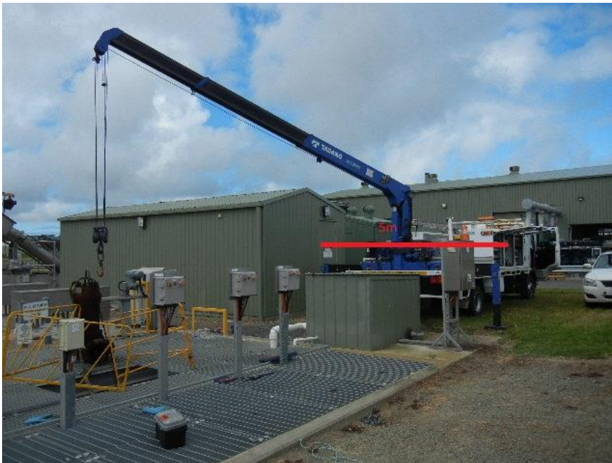
Figure 1: Crane Truck with Outriggers
